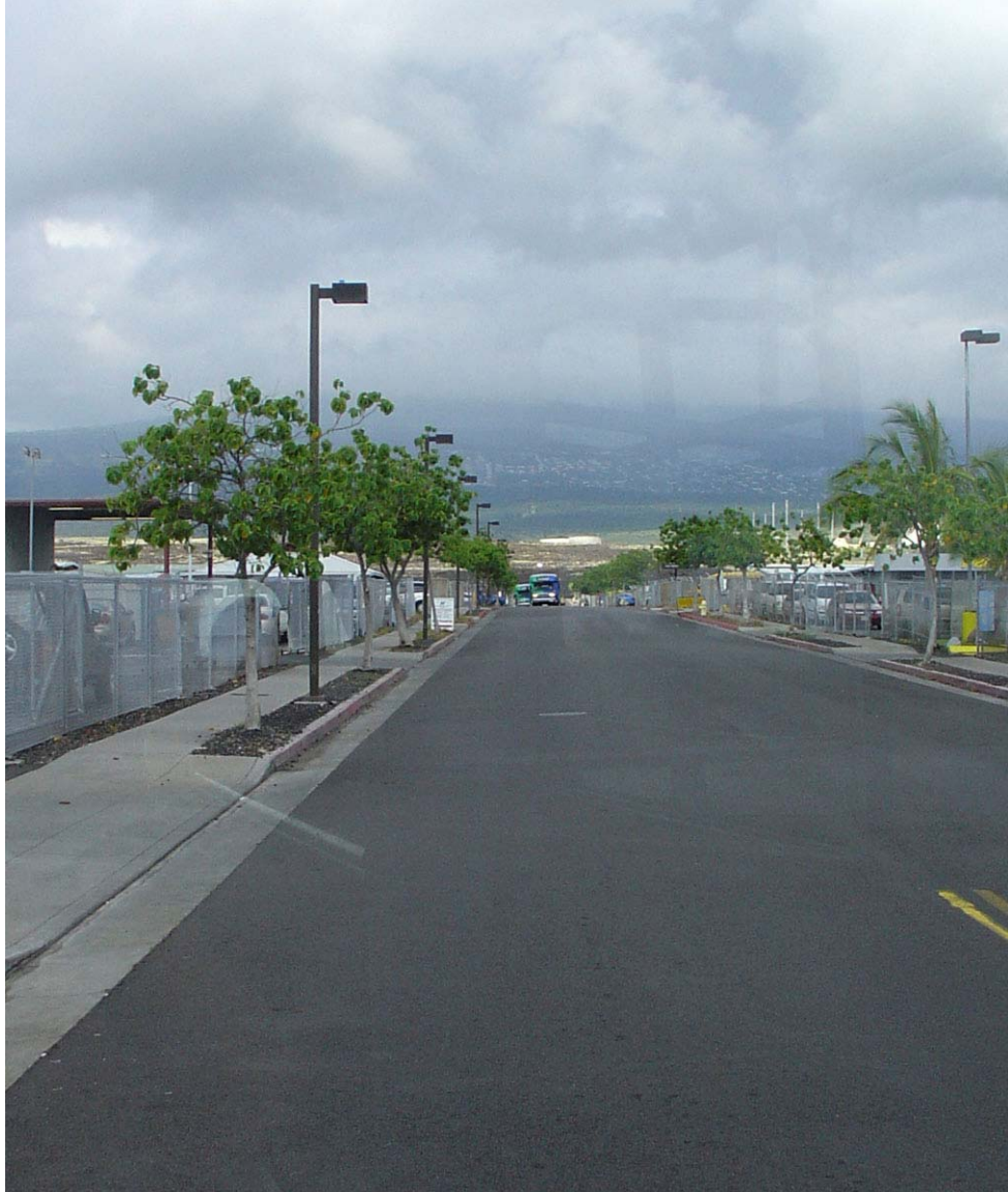
Newly installed lighting on the roadway at Kona airport near the car rental lots. These lights are high-pressure sodium. The Hawaii county lighting ordinance requires use of low-pressure sodium lamps for roadways.
