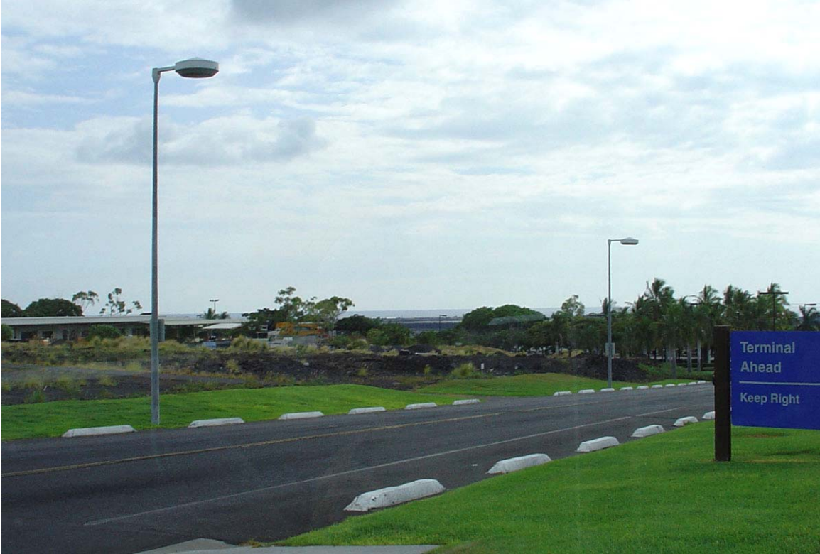
High-pressure sodium lamps along the access road to the Kona airport. The Hawaii county lighting ordinance requires use of low-pressure sodium lamps on roadways.
