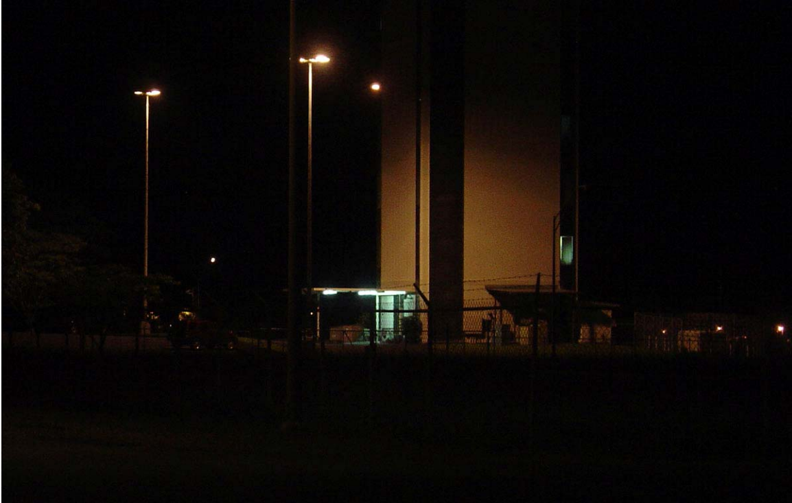
Lighting around the control tower at Hilo airport uses high-pressure sodium lamps. The Hawaii county ordinance requires that low-pressure sodium lamps be used on roadways.
